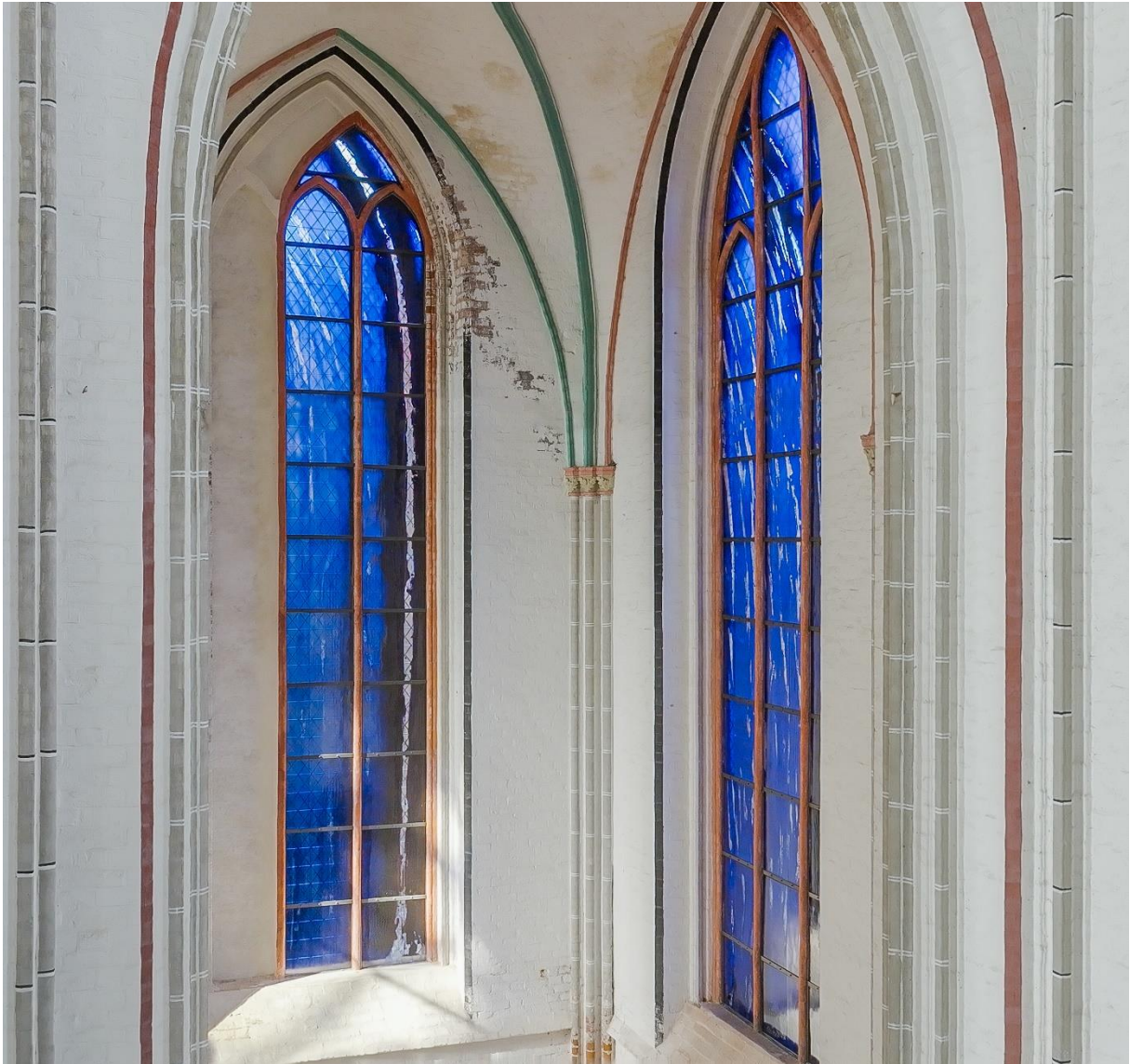
Completed Uecker-windows in the north-west section of the transept of Schwerin Cathedral. Copyright: Udo Tanske/Domförderkreis e.V.
